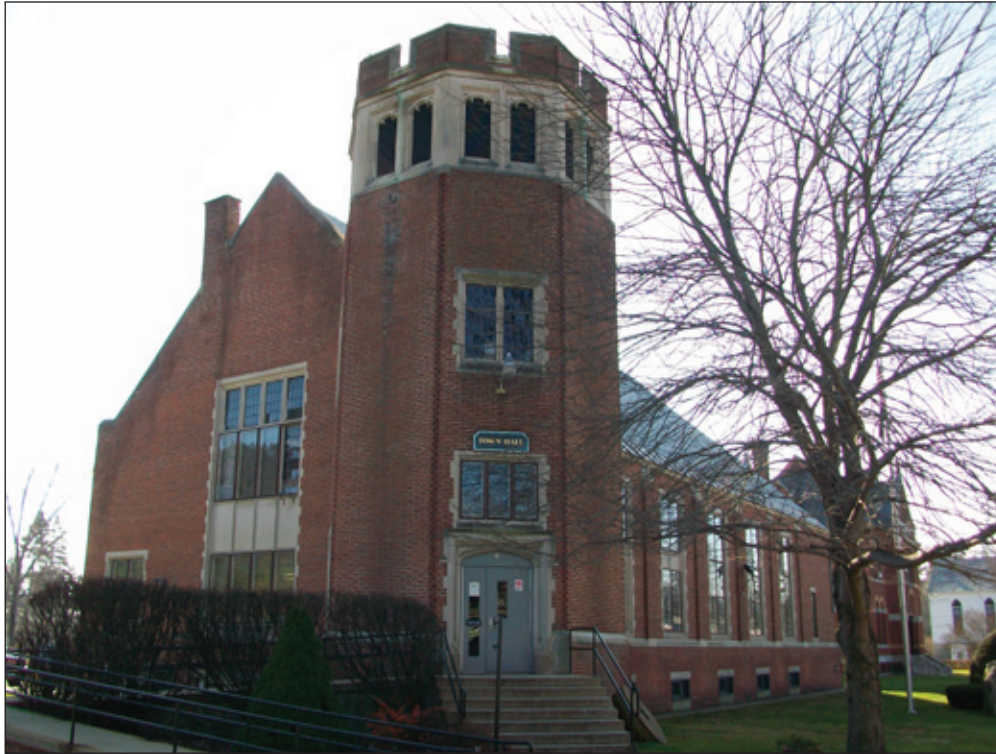
Winchester Town Hall. Photo courtesy of Dave Campbell.
